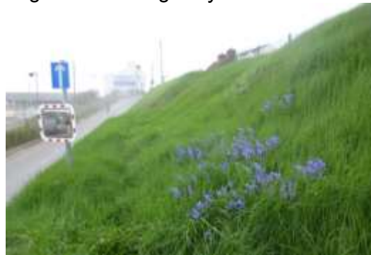
Basin Road North embankment
